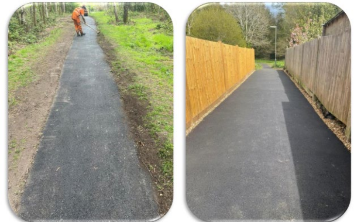
Figure 3: NE32 – Resurfacing of footpath between Hatch Gardens across Burgh Heath
